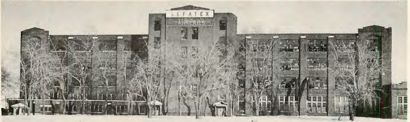
Building to be demolished is 250 feet long and 150 feet wide. Center elevator shaft is 120 feet high.
